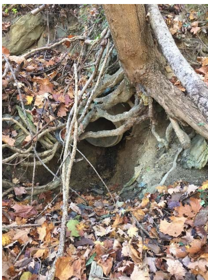
Failing concrete pipe
